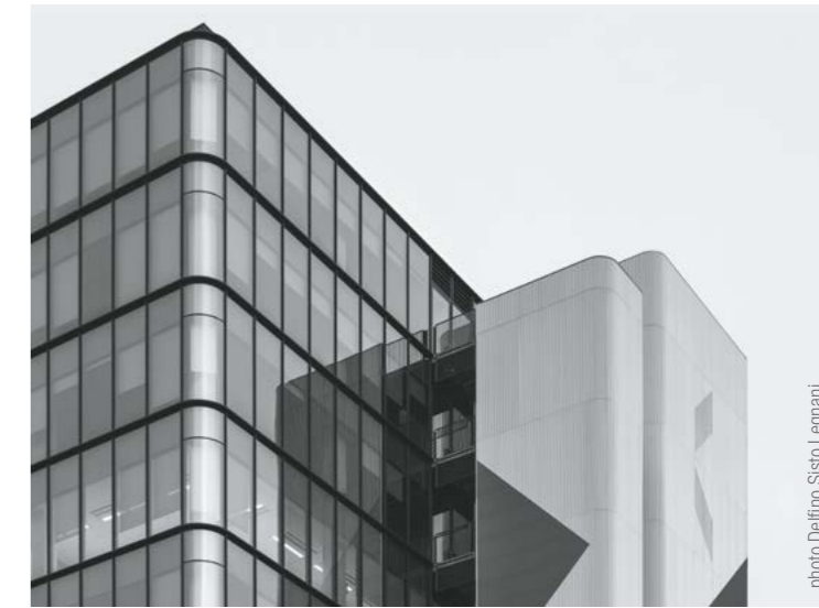
Sarca 235, office building in Viale Sarca, Milan, Italy.
